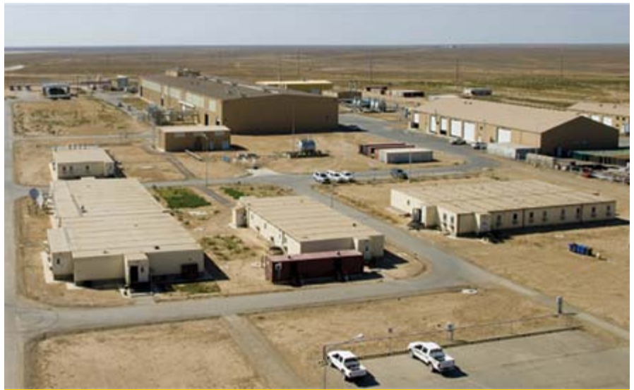
Main processing plant
